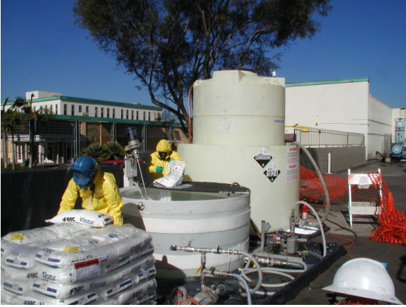
FIGURE 4. Mixing of persulfate solution.
