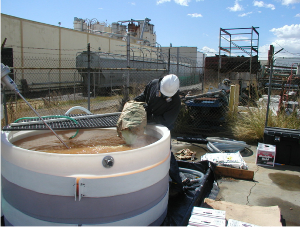
FIGURE 6. Mixing of ferrous sulfate into solution.
